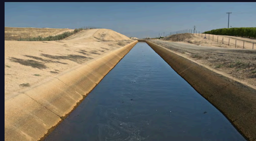
Oil slick on irrigation canal
