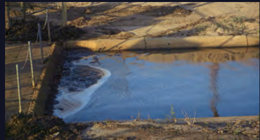
Oil waste build up at Cawelo intake
