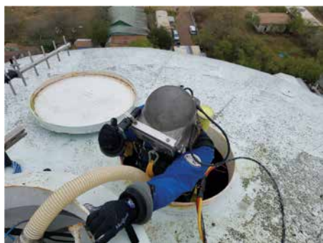
Diver entering Potable Water Storage tank. © Ron Perrin 2019
