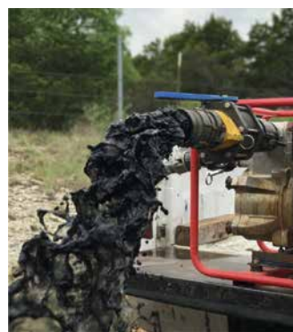
Sediment Being Removed from Potable Water Storage Tower. © Ron Perrin 2017-2019
