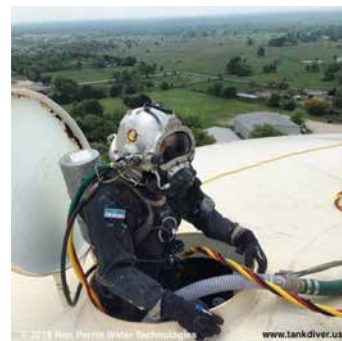
Diver entering Potable Water Storage tank. © Ron Perrin 2015-2019
