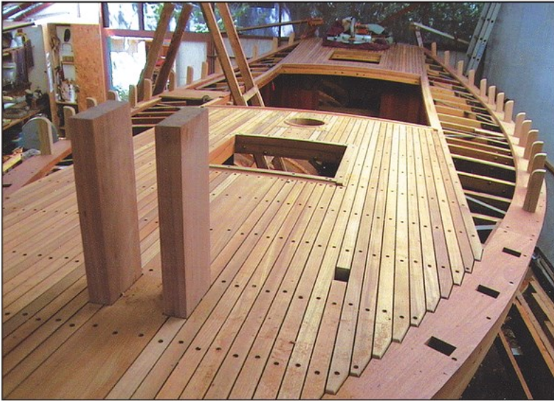
The teak deck planks are fit into nibbed covering boards, which are carefully mortised to receive the bulwark stanchions.
